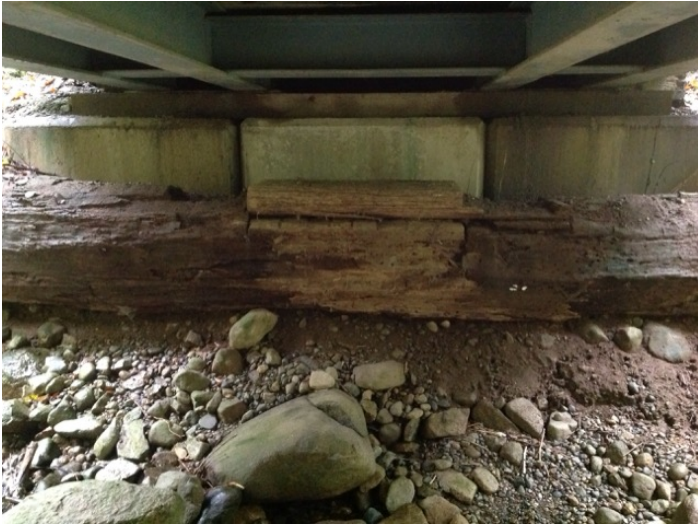
Left Bank Abutment when facing downstream
