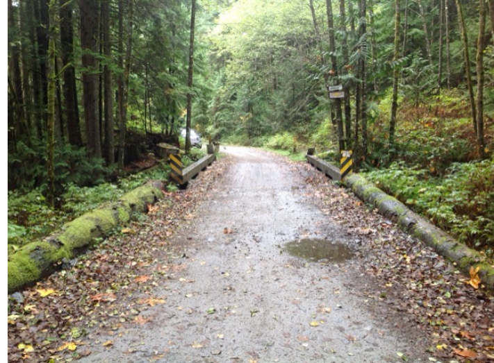
Approach from Left Bank when facing downstream
