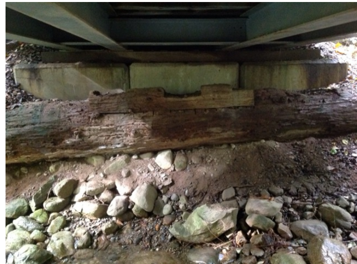
Right Bank Abutment when facing downstream
